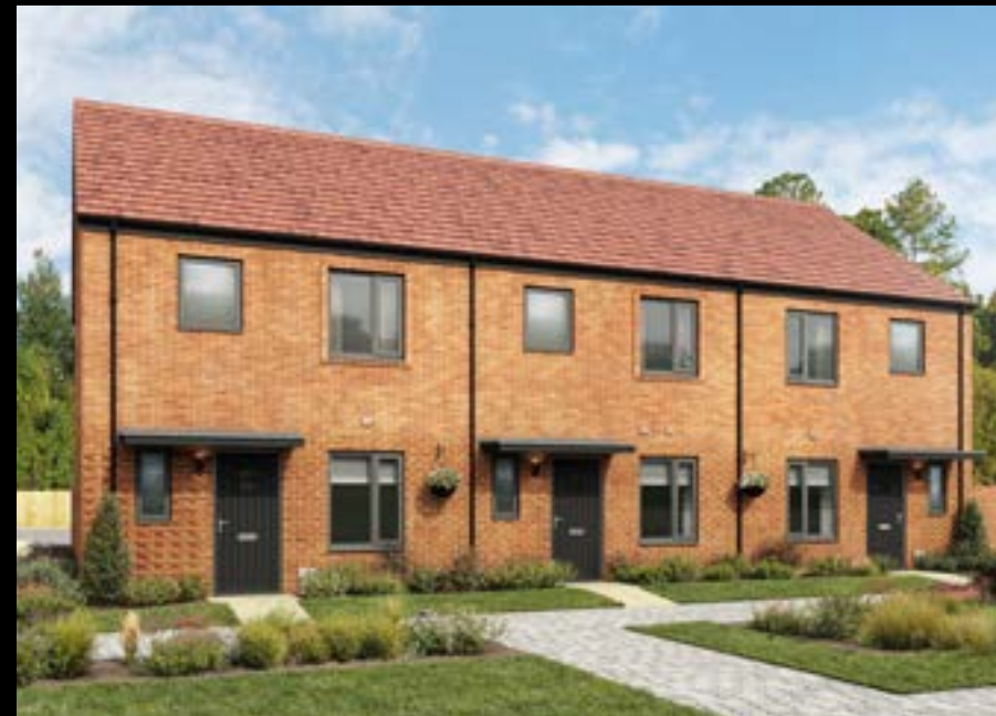
The Bayberry 2 bedroom semi-detached home and terraced home
