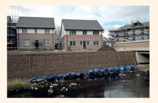
This system ensures surface water is dealt with sustainably via filter trenches, a series of attenuation tanks and a hydro break manhole system, which treats surface water run-off for diffuse pollutants while also providing storage to limit the discharge of it, thus ensuring the Water of Leith and its ecology are not impacted.
